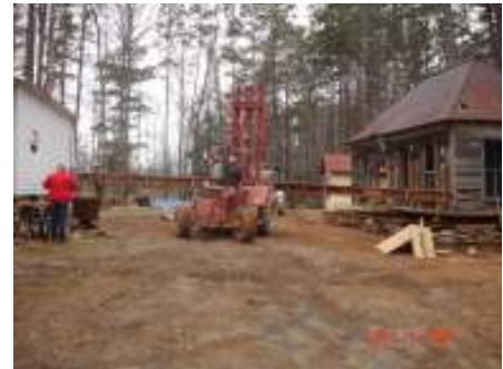
Steel girders on the way out!
