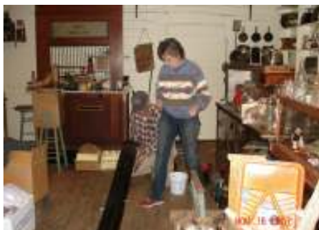
Charlie Burdick and Becky Griffin reposition the stove and pipe during improvements.
